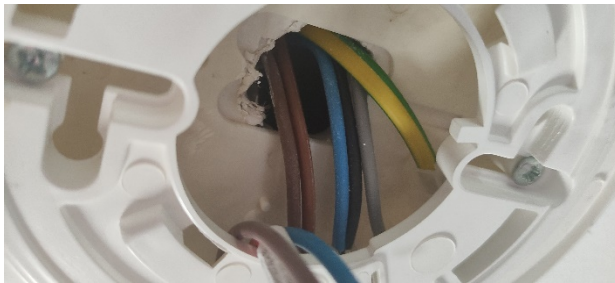
Hall (power 2 core + earth and to kitchen 3 core + earth)
